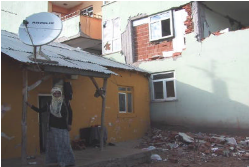
Figure 2. In Central Bingöl, life in a one story house adjacent to a heavily damaged high rise building (Photo: A. Nuray Karanci)
