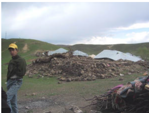
Picture 6. Cimenli Neighborhood /Village, one of the collapsed stone buildings (Photo by A. Nuray Karanci)
