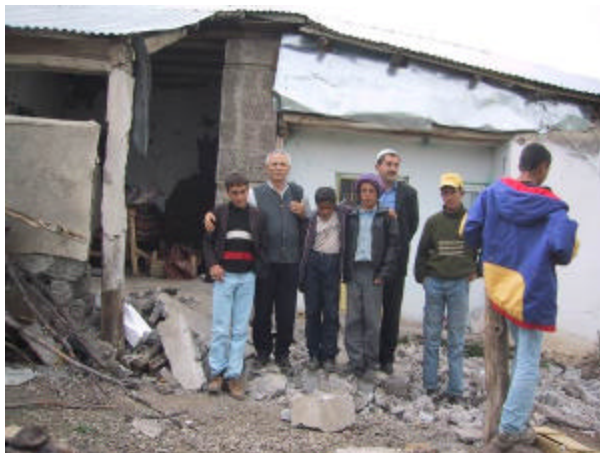
Picture 7. A group of children with the imam and a member from our team standing in front of the imam's heavily damaged house annexed to the mosque. (Photo by A. Nuray Karanci)
